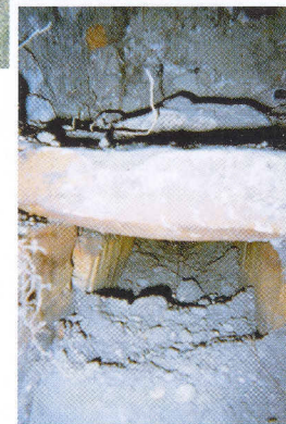
The conduit was an oblong construction, made of clunch blocks on the walls and roof, and was partially filled with grey silt. Orange staining of the stone surfaces inside suggested a waterflow in the past.
